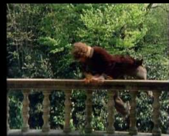
Hercules Hall balustrade
